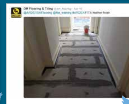
Michael Atkinson Flooring ARDITEX NA, a trusted favourite for years, ticks all the boxes! Applying over traditional victorian tiled floor which has adhesive residues, very slight movement in some tiles and no dpc. Overlaying with engineered oak plank.
