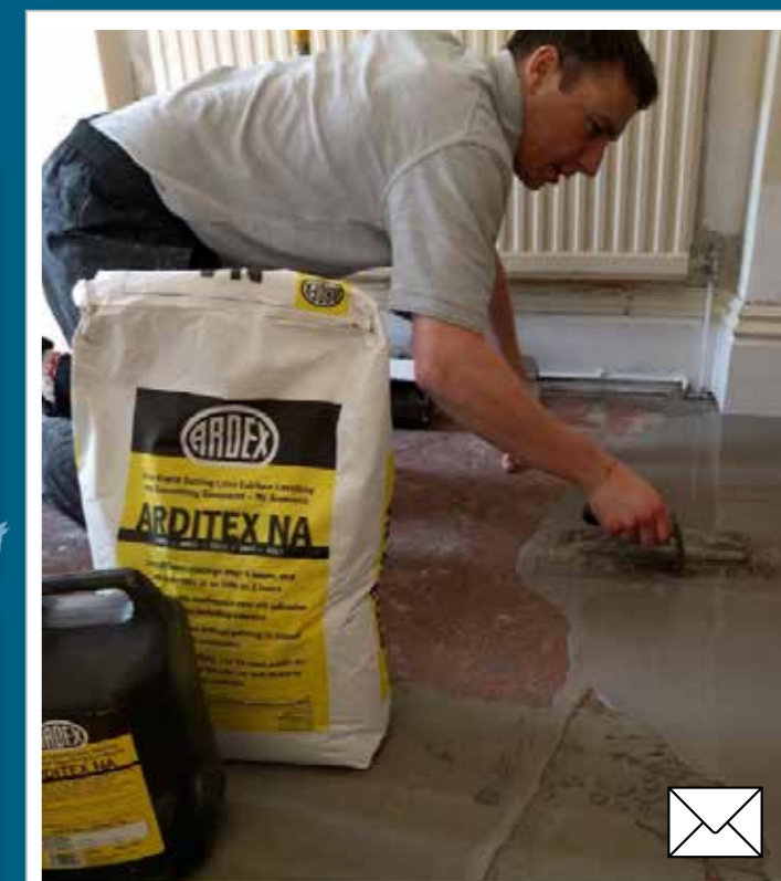
Michael Atkinson Flooring ARDITEX NA, a trusted favourite for years, ticks all the boxes! Applying over traditional victorian tiled floor which has adhesive residues, very slight movement in some tiles and no dpc. Overlaying with engineered oak plank.
