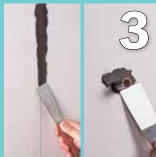
3 Apply the mixed ARDEX WPC with a spatula, pallet knife or trowel
