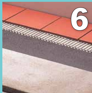
6 Finished installation. Tile on after 90 minutes
