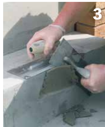
Shape hardened ARDEX A 46 mortar to the correct profile
