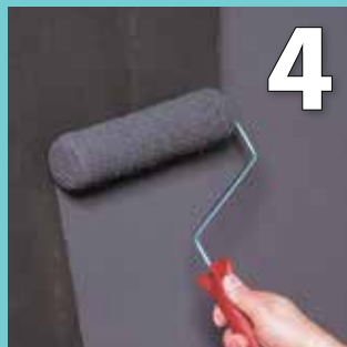
4 MIX 2: Mix to a flowing consistency. Apply an even coat with a paint brush or roller 30 minutes after the first coat
