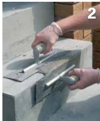
Apply ARDEX A 46 mortar
