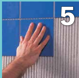
5 Tiles can be fixed onto the second coat after approximately 60 minutes
