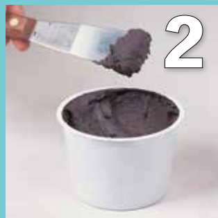
2 MIX 1: Mix a small amount of ARDEX WPC to a slump free consistency
